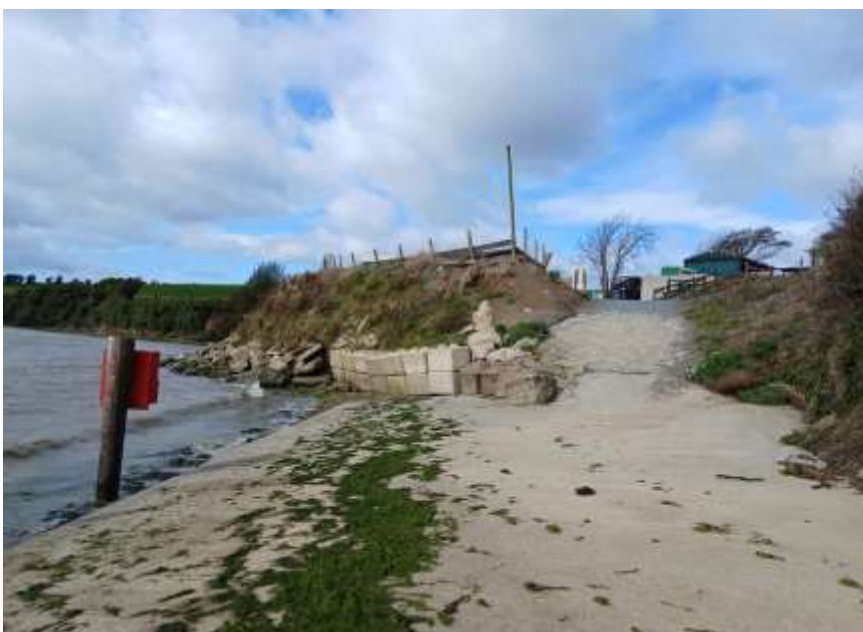
View from shoreline at jetty towards area of infill which is now used for campervan parking (fill material appears to largely be C&D waste material)
