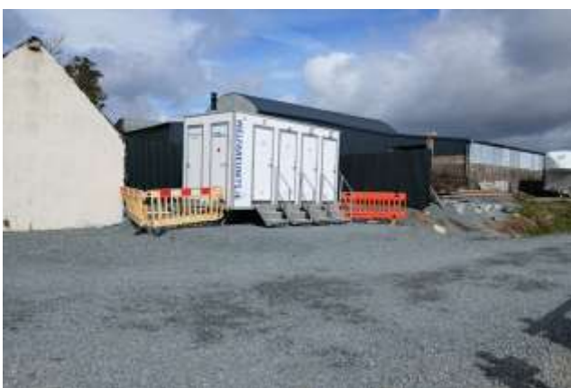
2no. welfare huts on site adjoining the farm sheds (chemical / hazardous waste is located to rear of blue portacabin). No information on where the waste from these welfare huts is being discharged or collection arrangements if applicable
